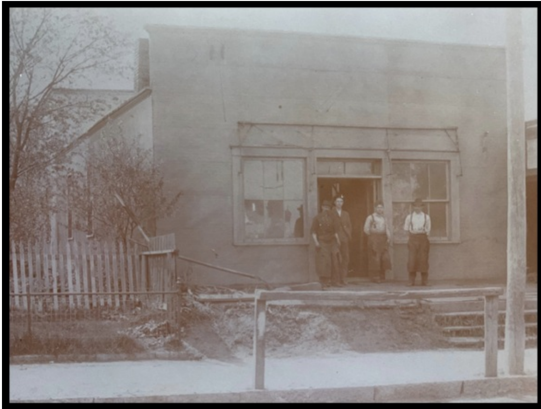
John March Blacksmith Shop on South Sampson Street
